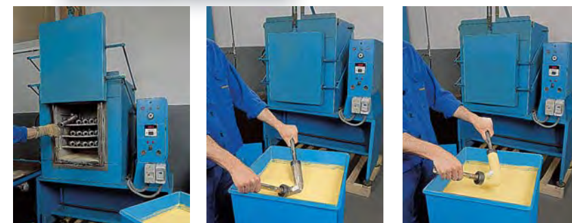
ANTICORROSIVE PLASTIC COATING
